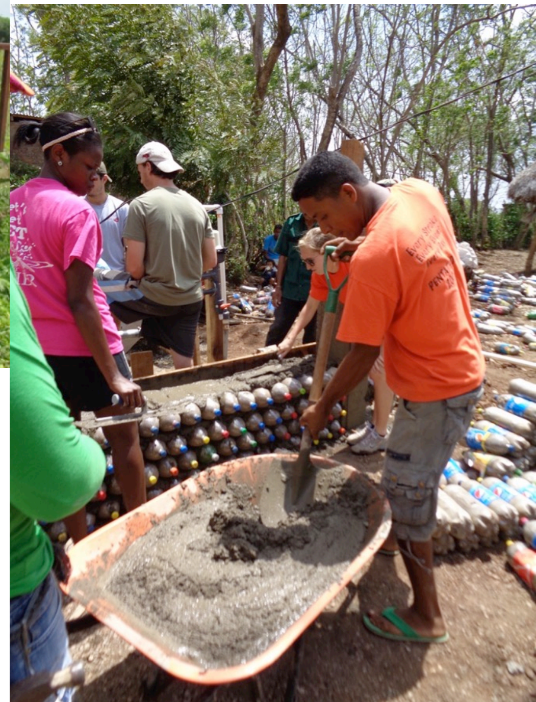
Constructing a certified hurricane-proof pump house out of recycled materials
