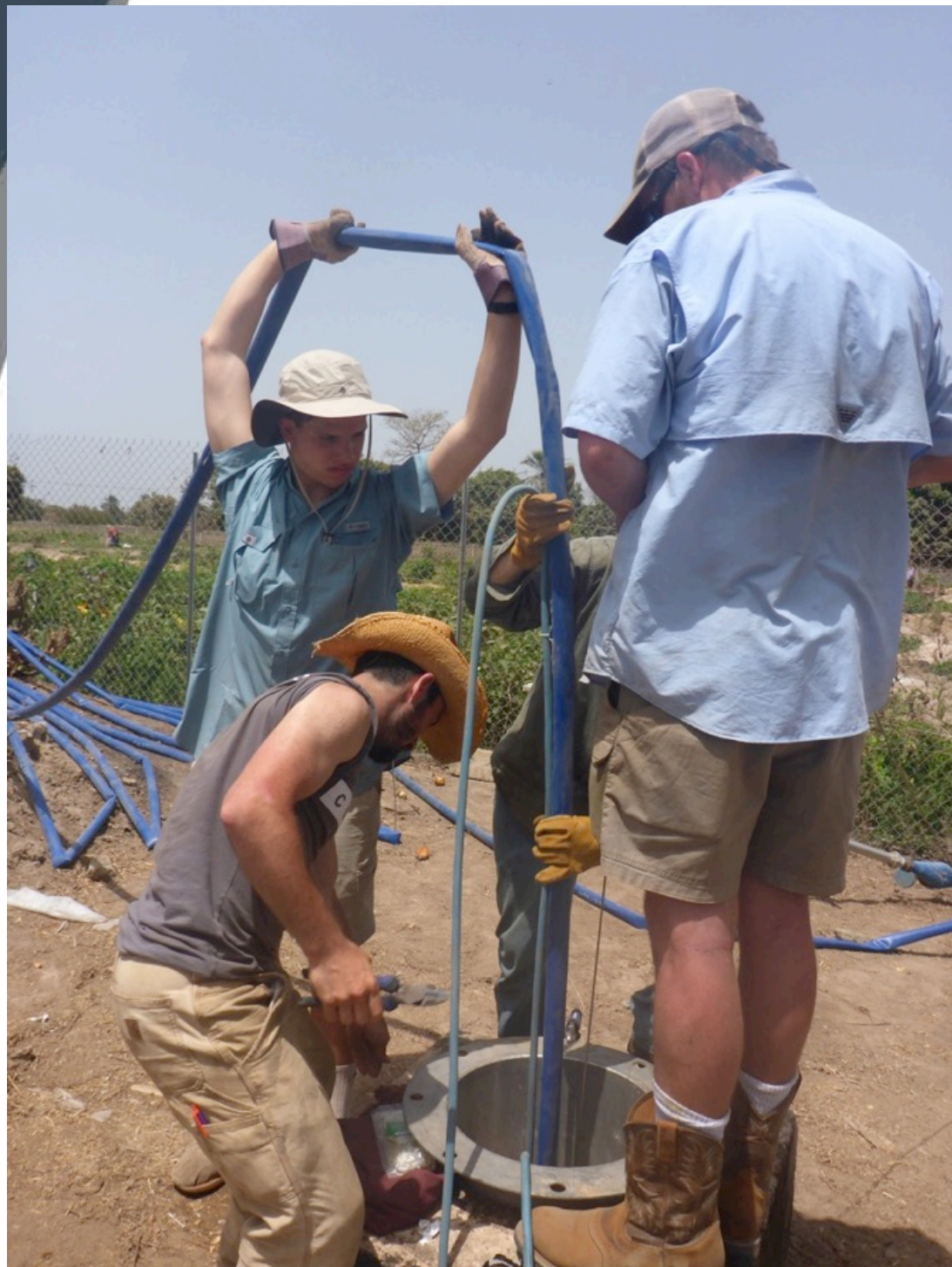
Performing well yield tests and repurposing solar panels from an abandoned well
